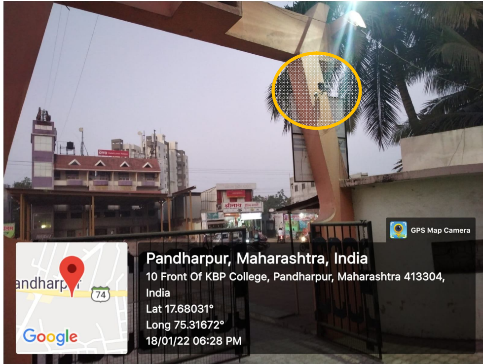
CCTV Surveillance at main entrance gate of college
