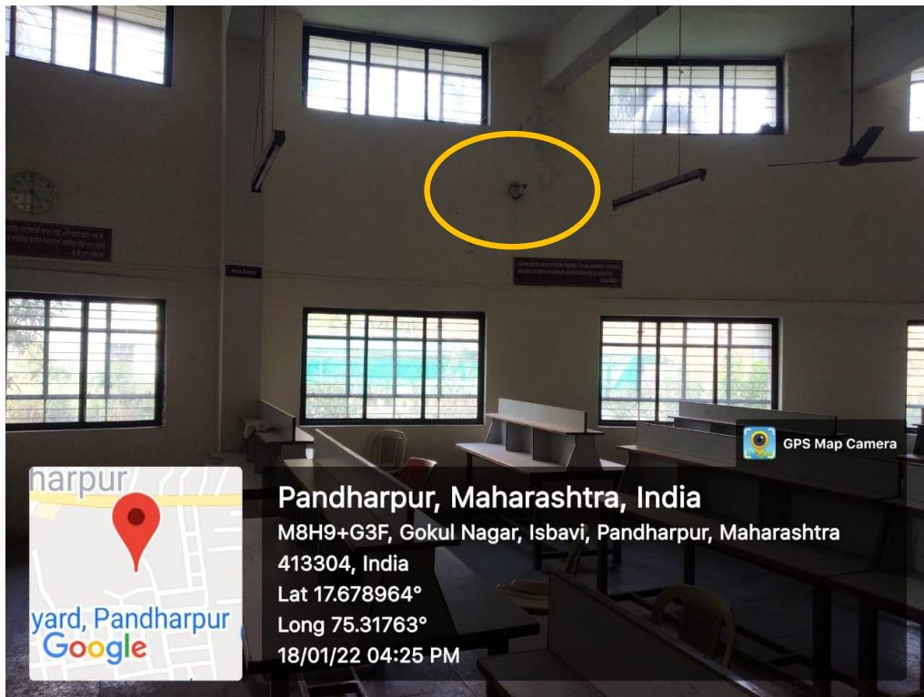
CCTV Surveillance at study centre in Central Library of college
